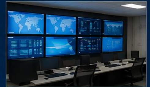
NETWORK OPERATIONS CENTER (NOC)
